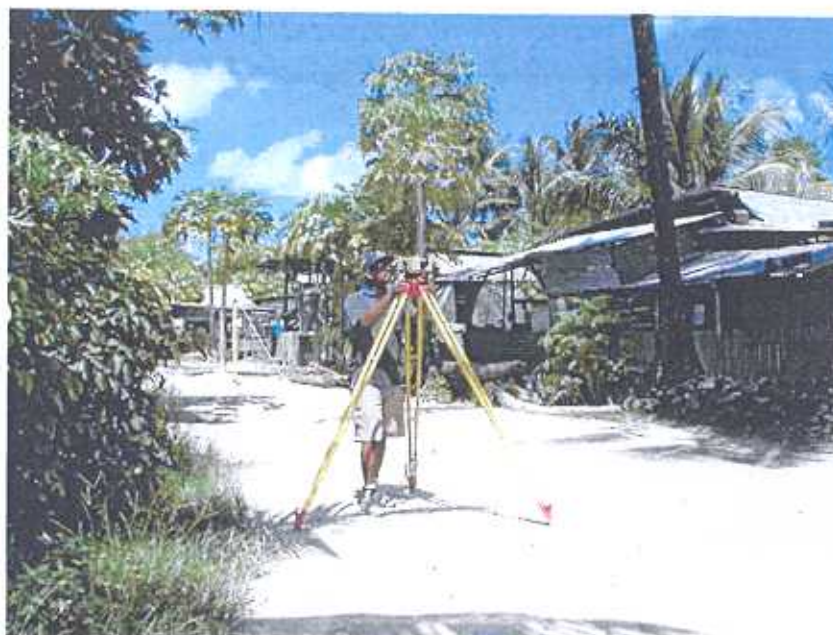
Levelling along road to the CGPS installation at the Meteorological Office.
